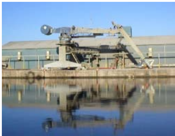
The 3.28m diameter upper and lower slew ring faces were machined flat and three pairs of badly worn link bore locations for the hydraulic lifting rams were rebored to accept new oversize pins.
